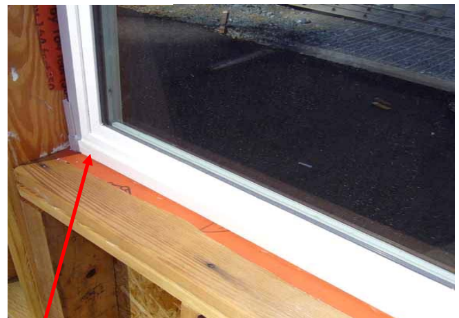
Sloped Sill Pan™ Installation Detail
