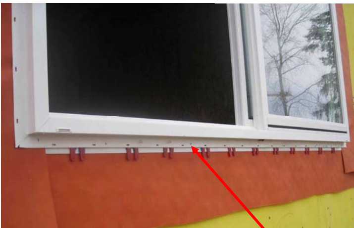
Sloped Sill Pan™ Installation Detail
